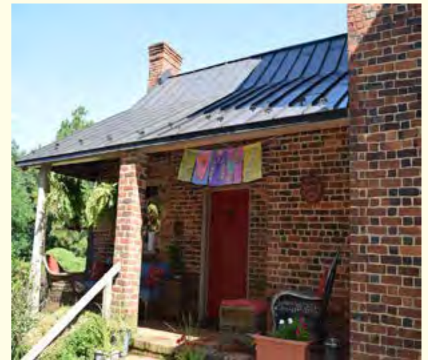
Rear of Charles Benbow House, Site #13
