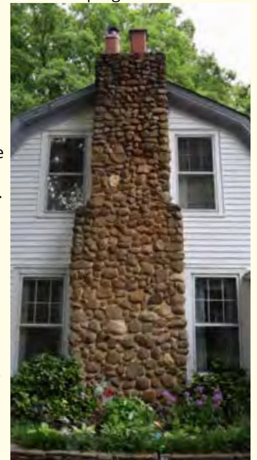
Stone Chimney at J.L. Sawyer House, Site #56
