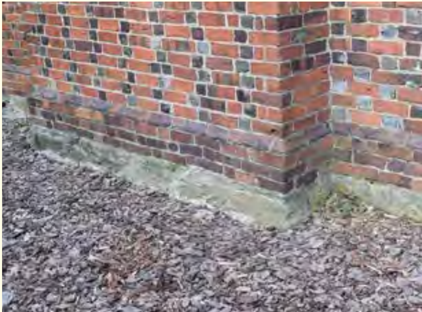
Foundation at Charles Benbow House, Site #13
