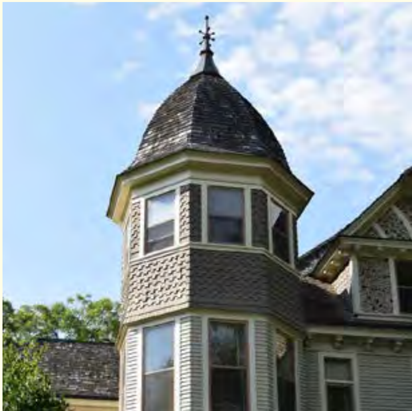
Roof on the turret at Oakhurst, Site #40
