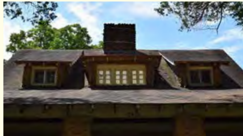
Dormered roof at D.L. Donnell House, Site #53
