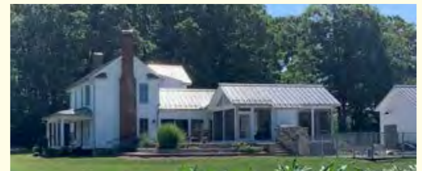
Relocation of Samuel Lowrey house on Pepper Rd.
