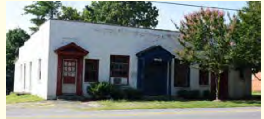
Flat roof at Holt Infirmary, Site #35b
