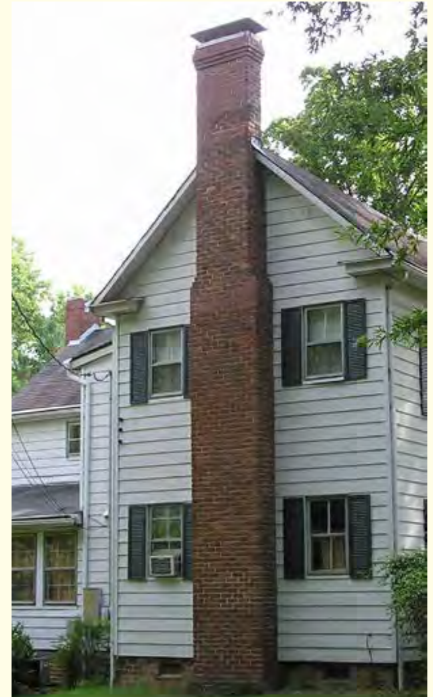
Brick chimney at Zack L. Whitaker House, Site #54
